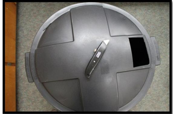
5. Carefully cut a hole in the lid of your rain barrel using the box cutter. This hole should sit under your home's downspout so the water runs directly into the barrel. Cut the hole so it's large enough to accommodate the water flow from the downspout.
