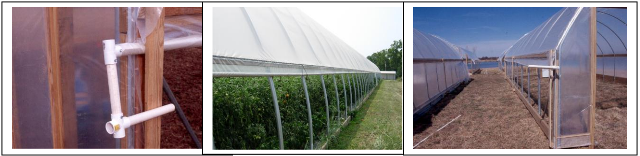
Figure 13. A L-shaped handle for rolling the sidewalls up or down.
