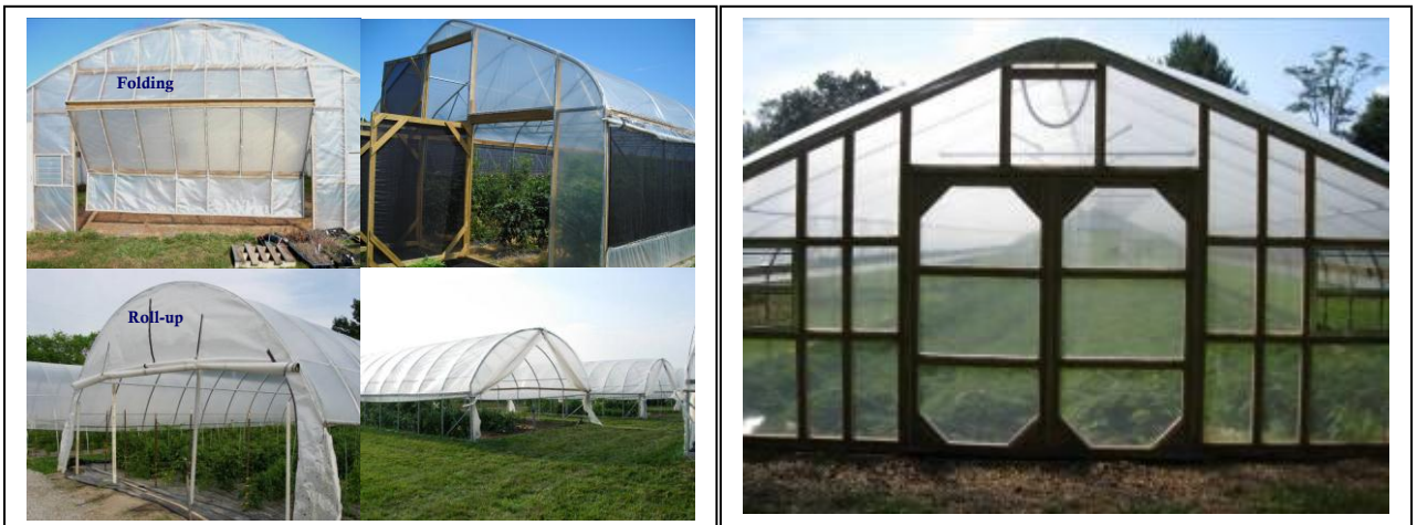
Figure 10. There is a diversity of end wall designs for high tunnel structures.
