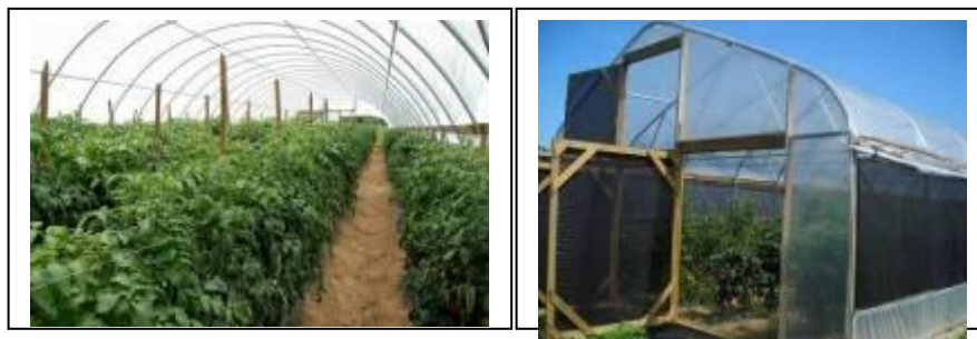
Figure 1. High tunnels are passively vented, solar greenhouse structures covered with a single or double layer of polyethylene plastic.
