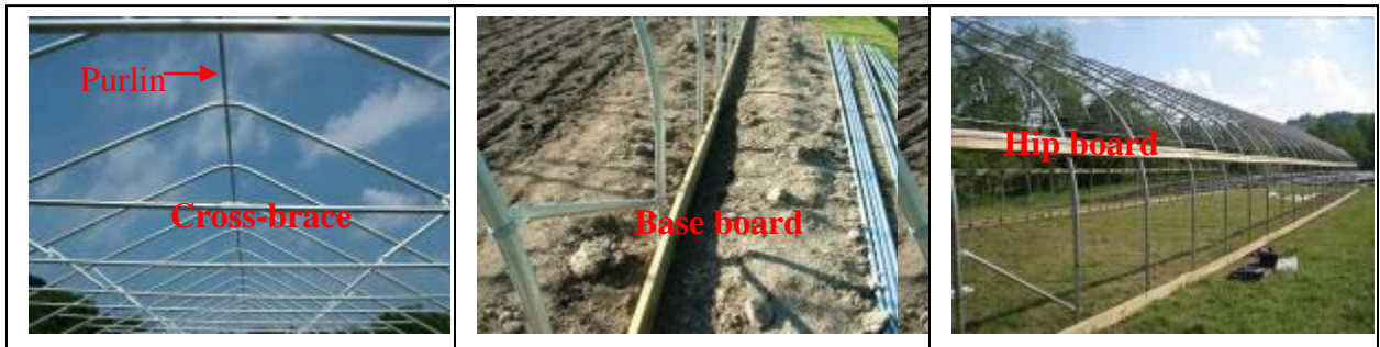
Figure 8. Purlins, cross braces, base boards and hip boards are attached to each bow to provide stability to the high tunnel frame.
