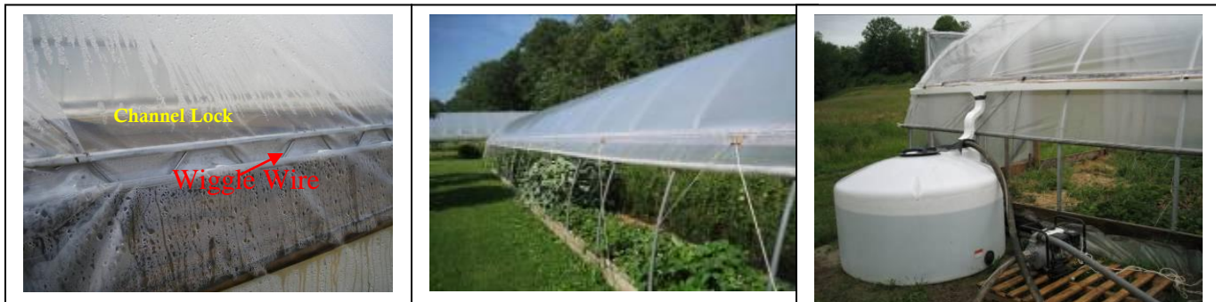
Figure 12. Plastic is secured to the frame with wiggle wire within each channel lock. Rope can be laced along the sidewall for tightening the roll-up sides. Water runoff from the high tunnel can be collected and used for irrigation.
